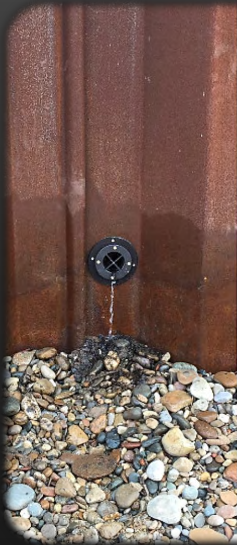
Steel Sheet Piling
